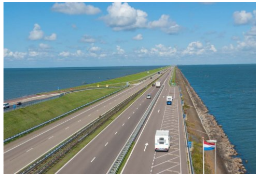
Figure 2: An actual dike
